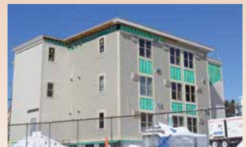
Jack's Place construction - April 2016
