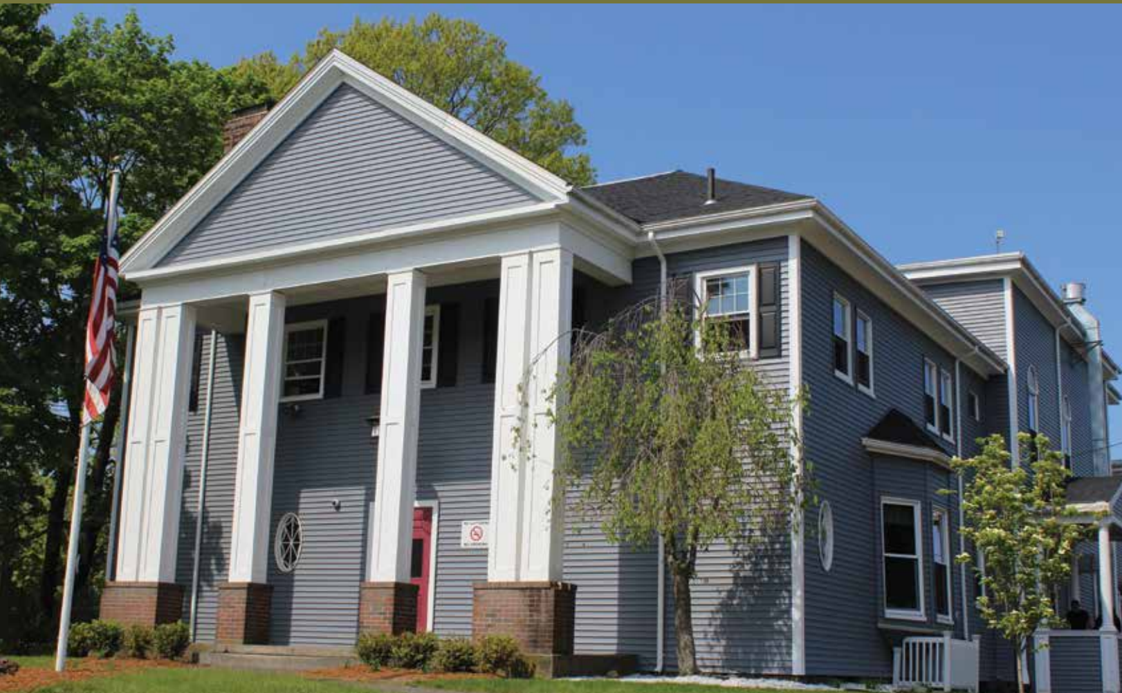
The MainSpring House emergency shelter in downtown Brockton has undergone some major renovations in recent years.
